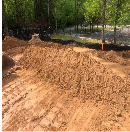
Building Pad Striping
