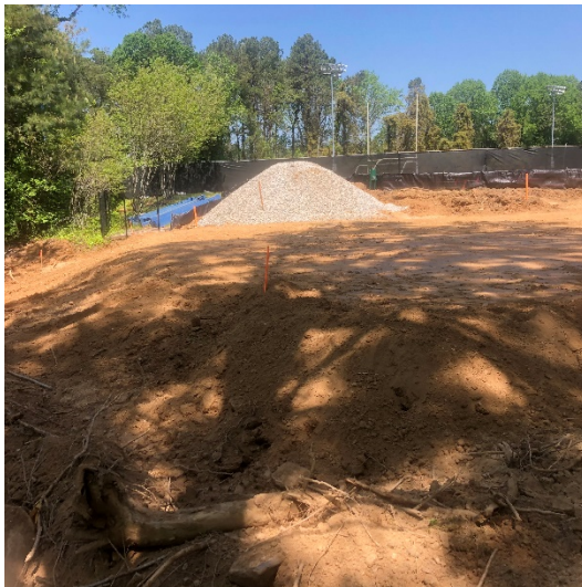
Building Pad Subgrade Prep
