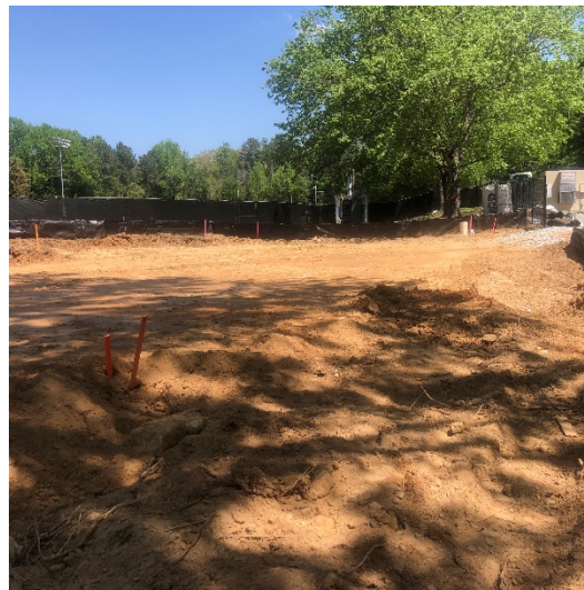
Building Pad Subgrade Prep
